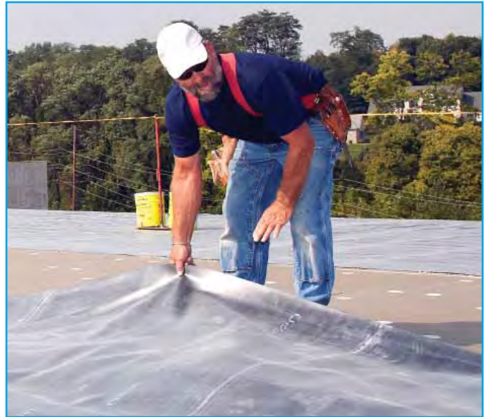
VersiGard EPDM with Quick-Applied Tape formats for wide-width sheeting includes a single-fold sheet.
